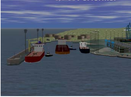
Figure 3 Oiltanking berth Marsaxlokk
